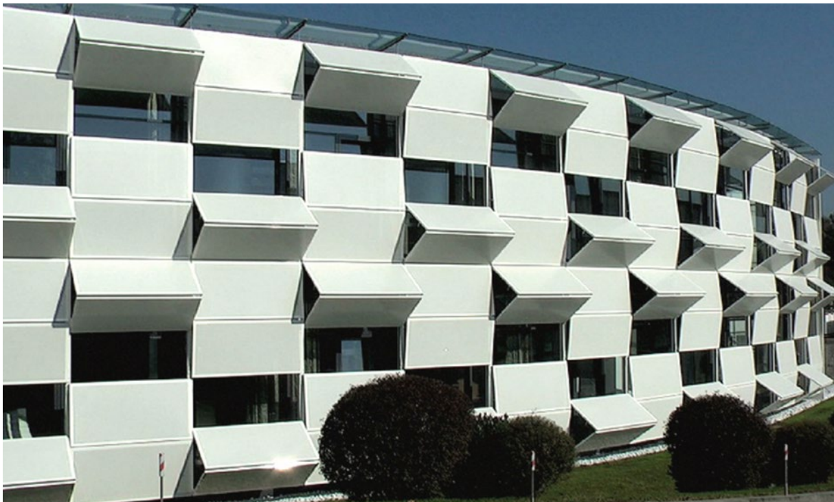
Figure 1-2 Kinetic shading façade of the Kiefer Technic Showroom.
