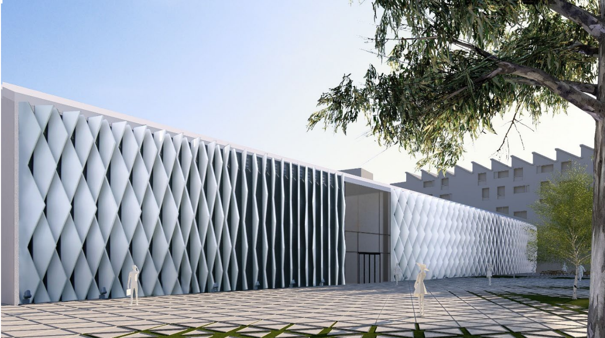
Figure 5-137 Rendered perspective view of the south façade with the optimized louver-based shading system.
