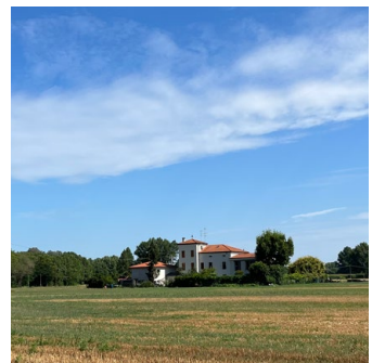
Figure 5.30 House in Use
