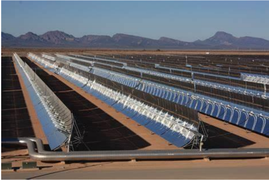
Figure 1-8 Solana solar plant in California.
