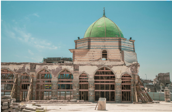
Fig. 5.2.2 The intervention for protecting destroyed Al Nouri Mosque.
