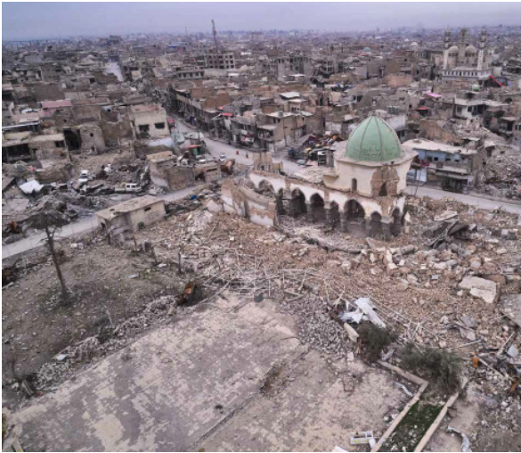
Fig. 1. 26 Drone View of Al Nouri Complex after its destruction
