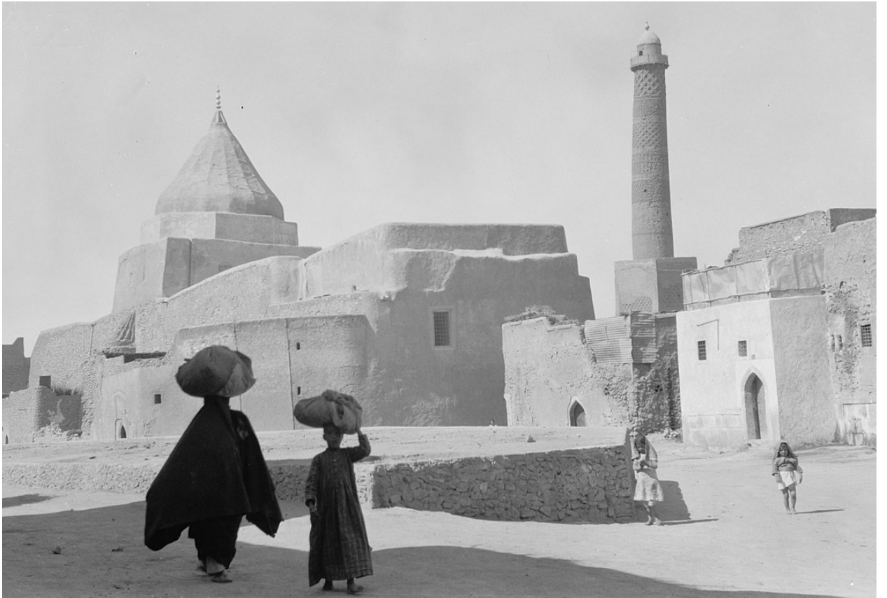
Fig. 3.38 The Mosque of al -Nuri with the al -Hadb ' Minaret, from the South-East, in its original state, i.e. before its demolition in 1942.
