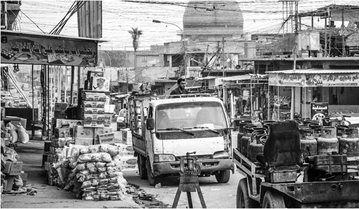
Fig. 3.25 Market street in West Mosul, Iraq, 2017, crowded street of the second category with a lot of commercial activities.
