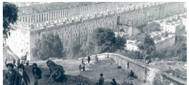
Fig. 4.67 general view of 200 columns
