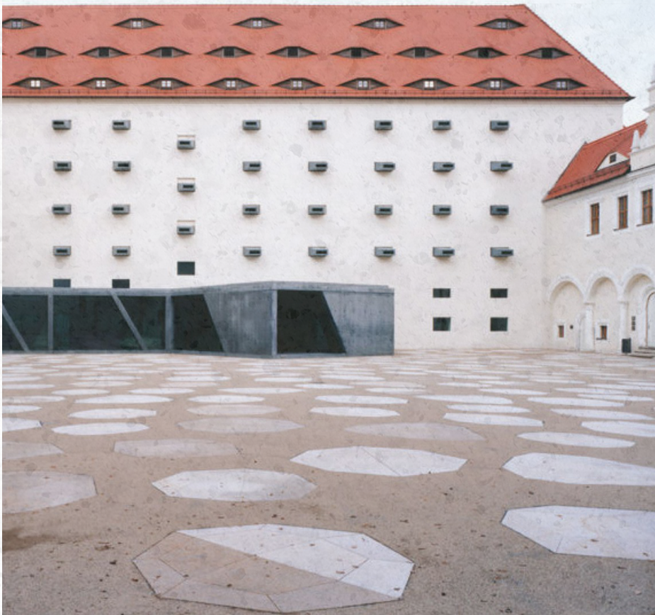
Freudenstein castle renovation, Freiberg 2010
