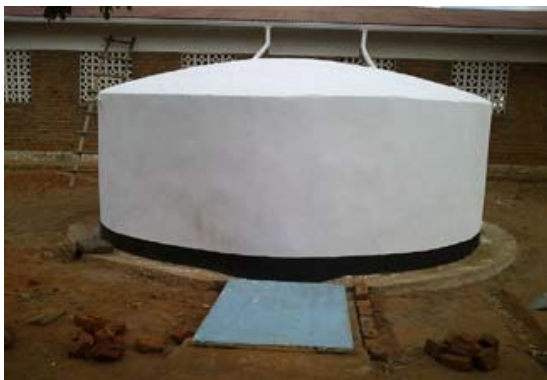
Figure 6-5 Above ground tank
