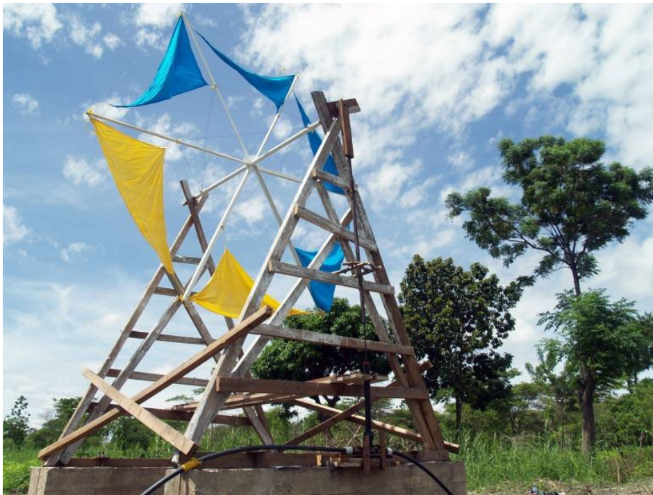
Figure 6-36 Wind pump construction
