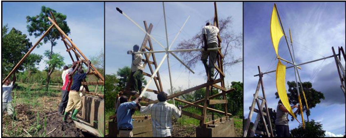
Figure 6-35 Wind pump construction
