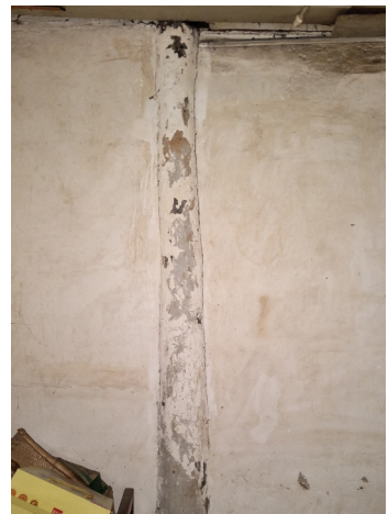
Fig. 5.24 Wood column visible in the interior of a local, the interior walls are thinner than the column
