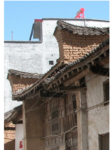
Fig. 5.26 A earth-bricks Matou Qiang, it's possible to notice the decoration made with roof tiles
