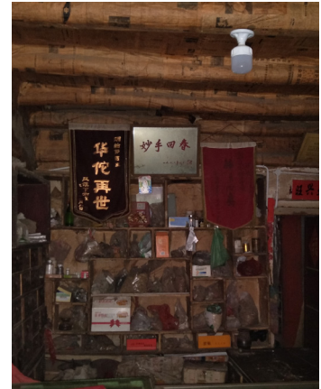
Fig. 5.31 Interior horizontal division, is possible to notice the presence of paper that was glued to the structure in order to protect it from humidity
