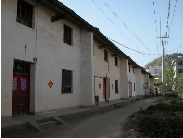
Fig. 5.12 Photo of a series of new buildings built with the ancient construction techniques, is possible to notice the Matou Qiang interpretation
