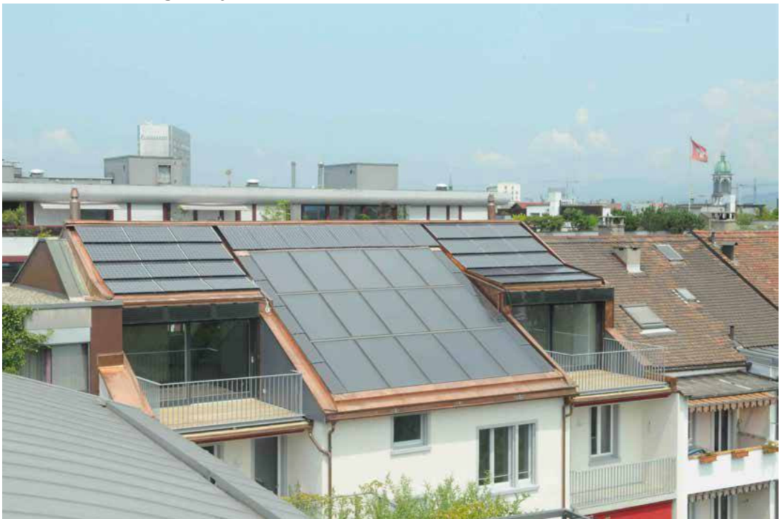
Fig. 3.11 Photo of the roof photovoltaic system, the two smaller pitches are used to produce hot water.
