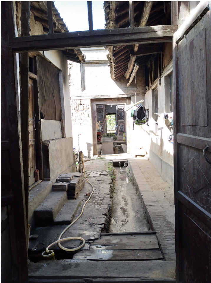
Fig. 5.8 Photo of a double courtyard is noticeable the impluvium that's present in the center of all the buildings that belongs to this category.
