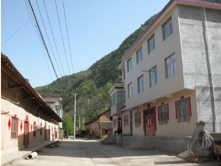
Fig. 5.16 Photo of modern buildings with a concrete structure
