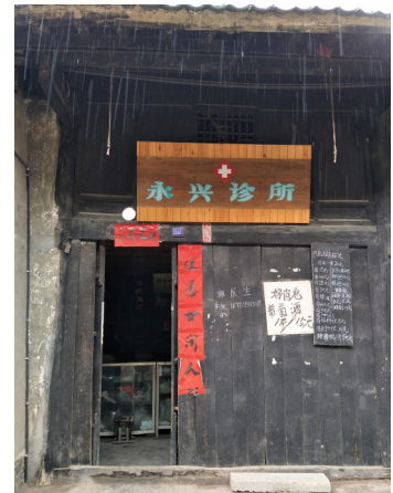
Fig. 5.32 Facade opening, the single wood planks are removable, allowing the resident to adapt the "door" to his needs
