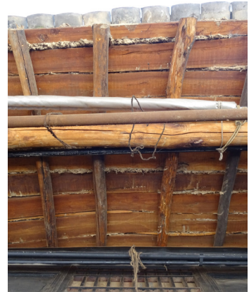
Fig. 5.29 Roof wood structure, it is possible to notice the rammed earth layers use to insulate the wood planks and also to offer sustain to the tiles
