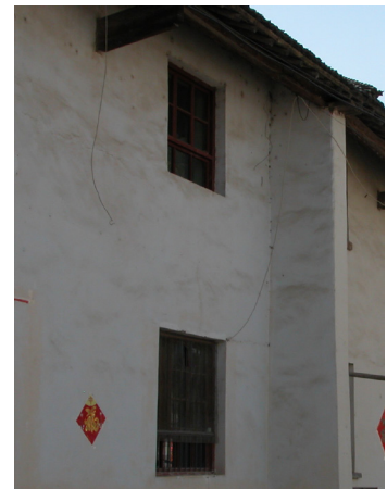
Fig. 5.35 Exterior walls of the typology, here is possible also to observe the different openings from the previous category and also the presence of a different type of Matou Qiang
