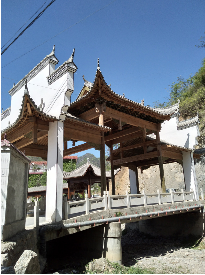
Fig. 5.21 Photo a bridge that was built on the river, imitating the ancient techniques, this solution creates false historic buildings
