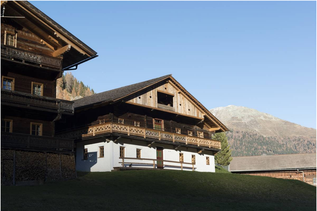
Fig. 3.2 Photo of the Giatla House after the restoration
