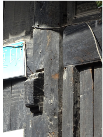
Fig. 5.23 Detail of the wooden beam on the facade
