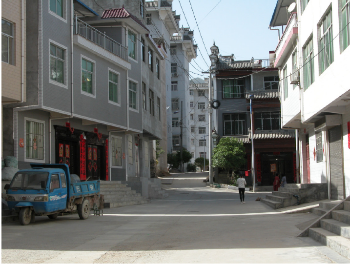
Fig. 5.15 Photo of modern buildings with a concrete structure
