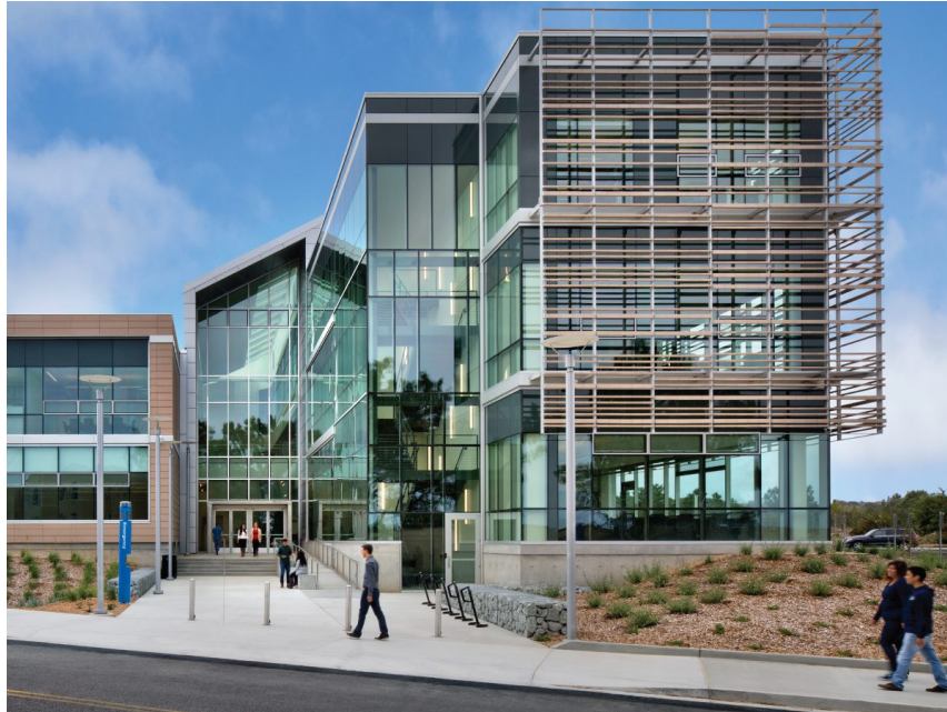
Figure 6: Exemplary Image for Irregular External Shading, The Joel and Dena Gambord Business and Information Technology Building, HMC Architects, California State University US [21]
