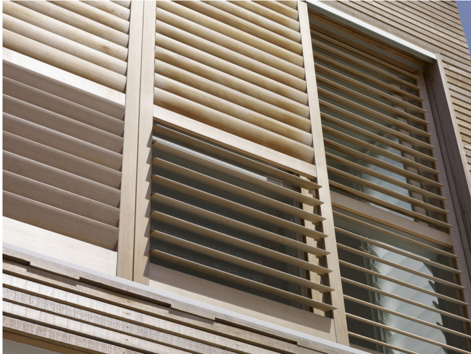
Figure 3: Exemplary image for Regular External Louvres, Thurston Elementary School, Malum Architects Inc., Oregon US [21]
