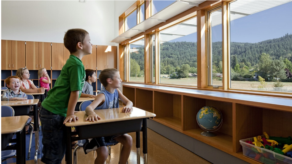
Figure 8: Exemplary Image for Light Shelf, Thurston Elementary School, Mahlum Architects Inc., Springfield, Oregon US [21]
