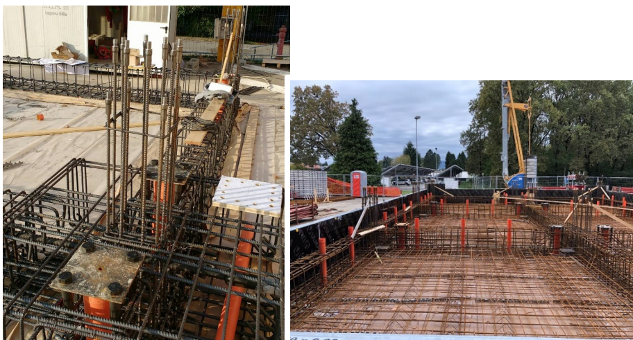
Figure 4.5 Rebars and plastic tubes detail.
