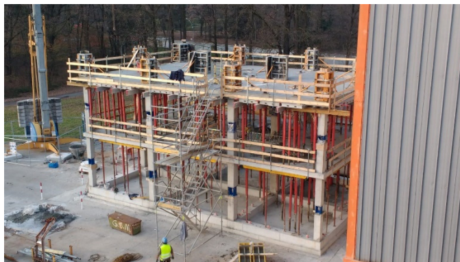
Figure 4.10 Props and safety measure for all the structure.
