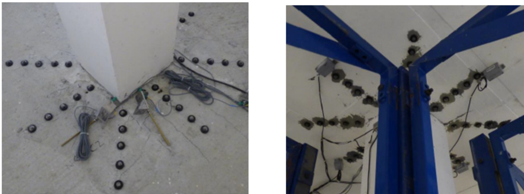
Figure 4.68 Repair of the central column on the 1 st floor.
