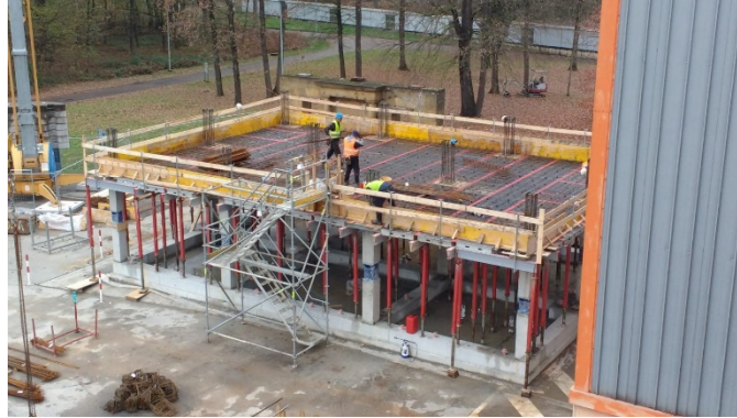
Figure 4.7 Placing of the formworks for casting the first floor.
