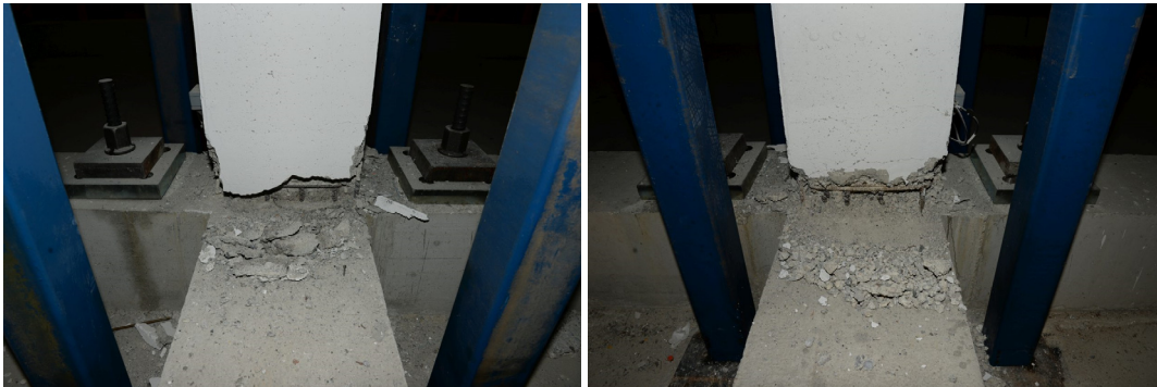
Figure 8.30 Base column connection B2 a) east and b) west, test Cyc-2 (g04).
