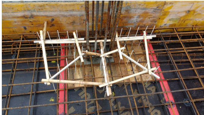
Figure 4.9 Plastic tubes positioning in the slab-column connections that will be strengthening.
