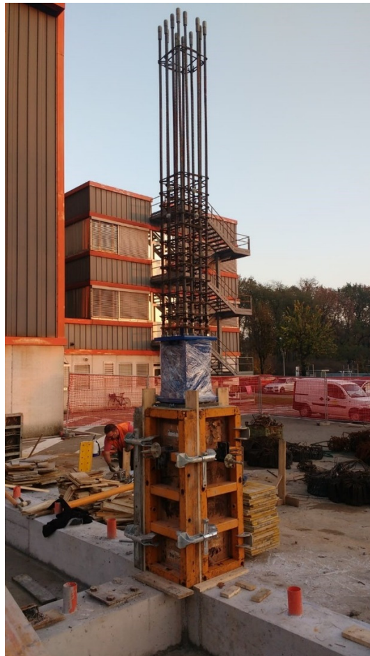
Figure 4.6 Column details: reinforcement, load cell and formwork.
