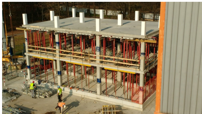
Figure 4.1 Construction of the specimen outside the laboratory.
