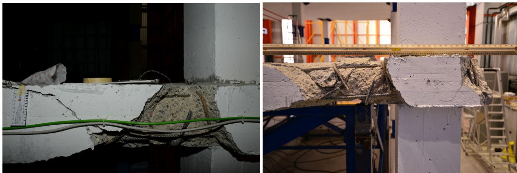
Figure 9.11 SlabSTRESS D1 east after test a) Cyc-1 and b) Cyc-2.
