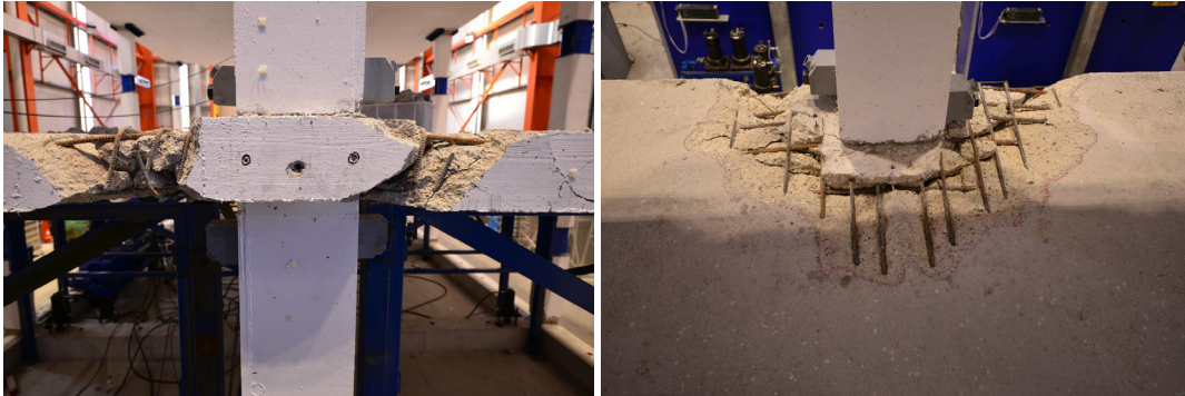
Figure 8.27 D2 connection after test Cyc-2 (g04), a) slab east side, b) slab-column connection.
