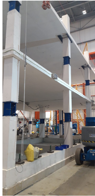
Figure 3.9 Steel stub in the columns.
