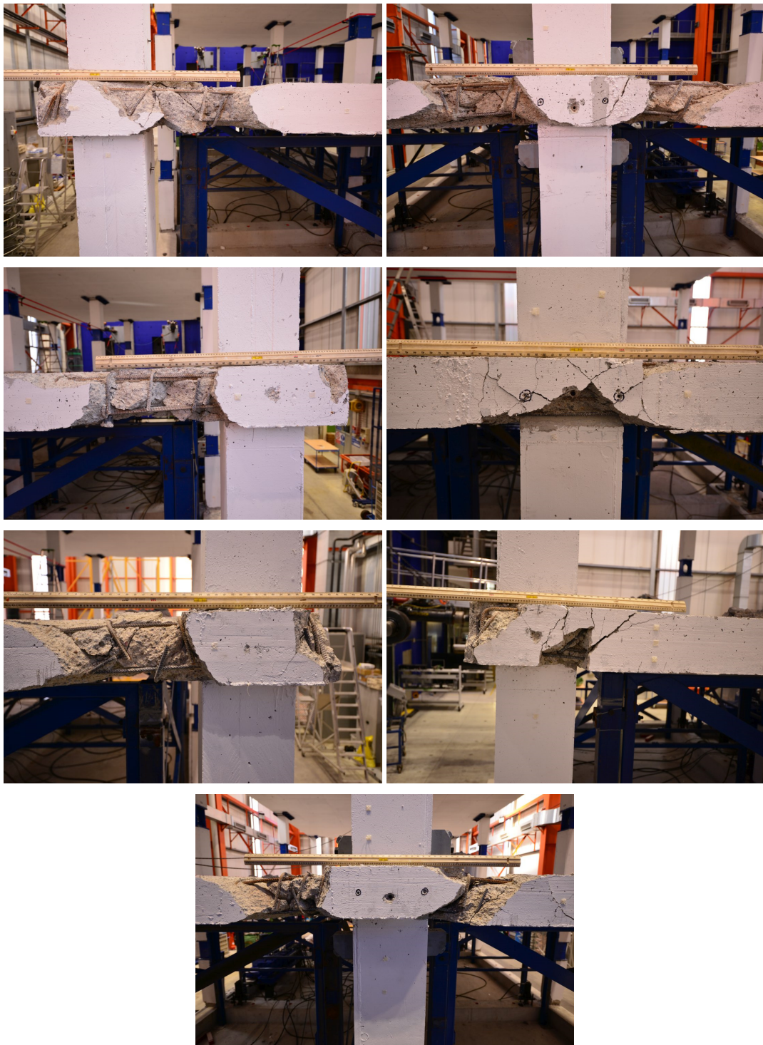
Figure 9.2 1 st floor slab edge damage, connections, clockwise direction a) A1, b) A2, c) A3, d) B1, e) D1 east, f) D1 north, g) D2 at the end of the experimental campaign.
