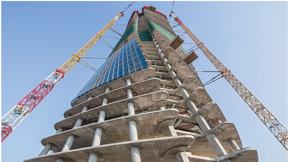
Figure 1.6 Example of flat-slab building in Milan [1]
